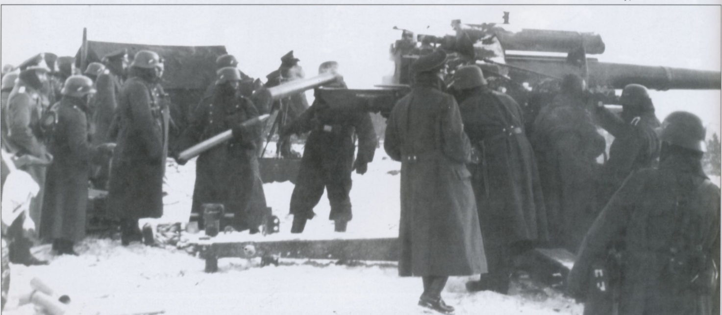
Third of the series showing the spent casing being ejected after firing. Loader stands ready with next round. The breech opened automatically via recoil or by hand. A good crew could fire between 12-15 rounds per minute (vertically or horizontally).
